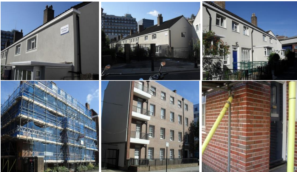
Figure 1: External wall insulation projects in Origin Housing stock
