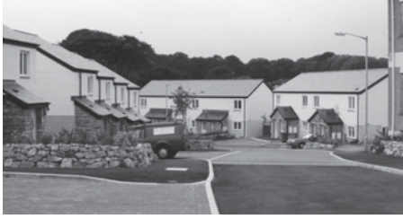
PENMERE CLOSE, PENWITH HOUSING ASSOCIATION, WAS BUILT ON THE SITE OF A FORMER SCHOOL KNOWN AS HUMPHRY DAVY
